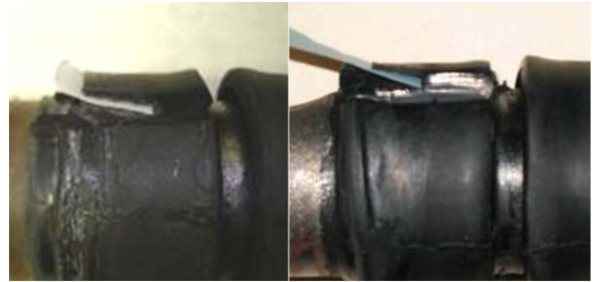
Figure 8: Crack Initiation from Field Test (left) and Lab Test (right)
